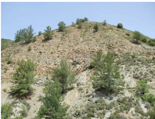
Photo 2. View of the Kakopetria detachment separating highly rotated, sub-horizontal dikes (top) from sheared gabbros (bottom) [Varga, 1991].
