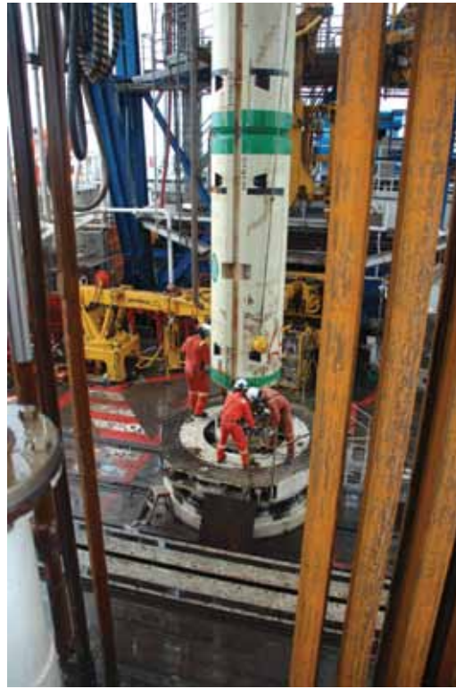
Figure 5.1. Rigging the riser during Chikyū operations for the Nankai Trough Seismogenic Experiment (NanTroSEIZE) in 2009. The Nankai subduction zone off the eastern coast of Japan has a 1400-year-long recorded history of magnitude 8+ earthquakes recurring about every 120 years. Riser drilling brings new capabilities to scientific ocean drilling, including downhole measurements of pore pressure and stress, and deep penetration in unstable formations to allow sampling of active fault zones. These measurements are enabling Earth scientists to gain a better understanding of how, when, and why great earthquakes occur. Photo courtesy of Y. Kano, Kyoto University.
